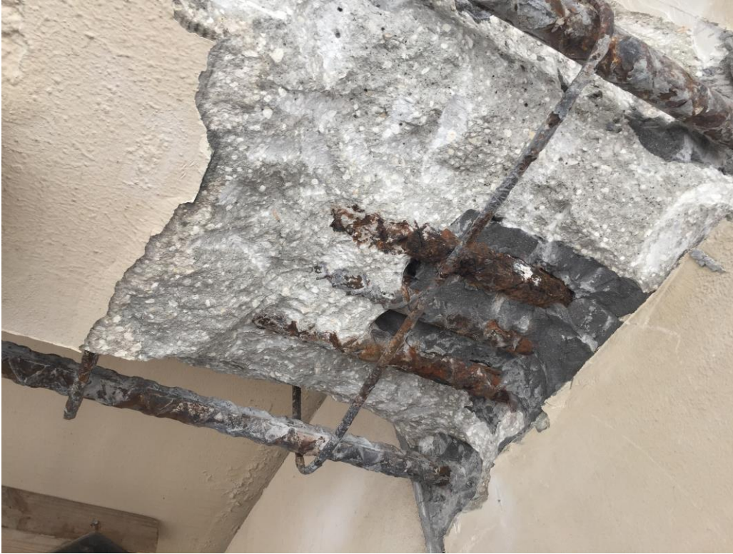
Picture 3: In-progress excavation
