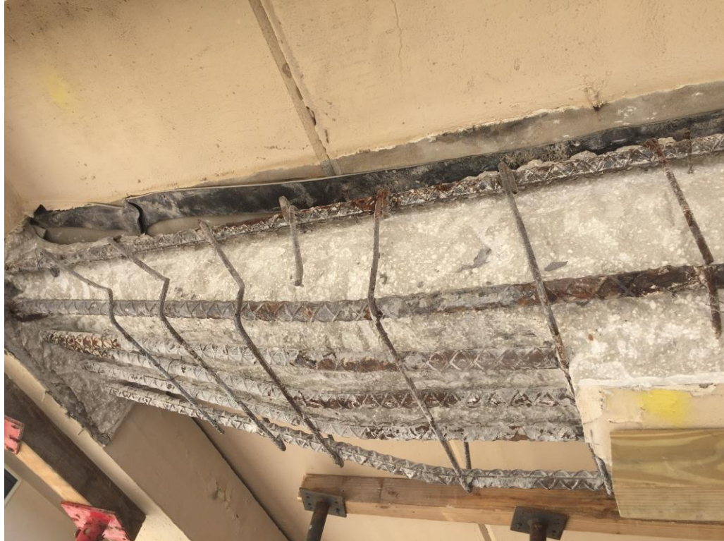
Picture 4: In-progress excavation
