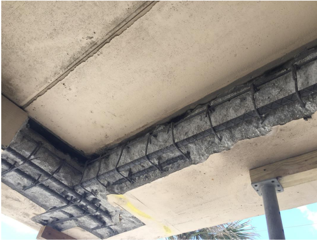
Picture 1: Typical beam excavation
