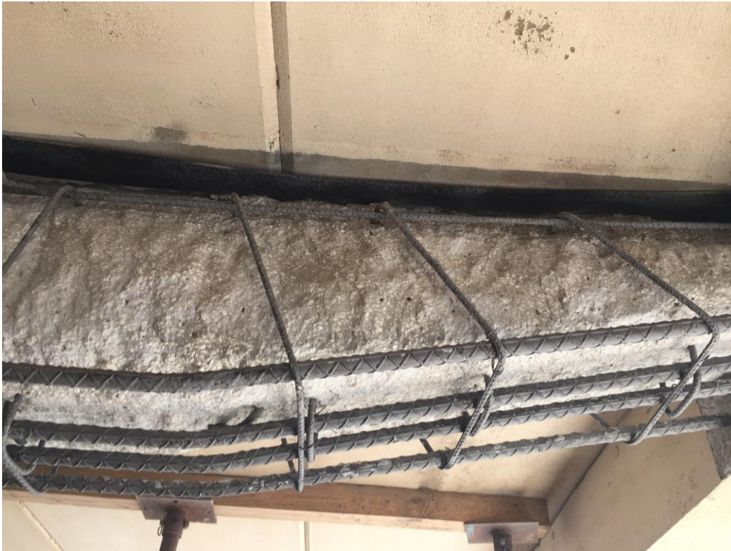
Picture 2: Typical beam excavation
